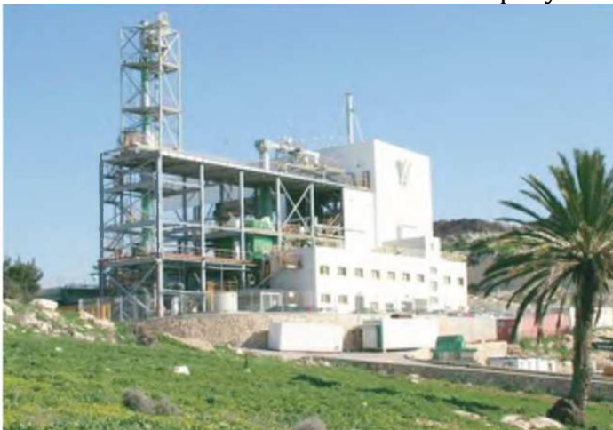
Fig. 2.21 – general view of the technological complex for the treatment of solid household waste in Israel [17]
