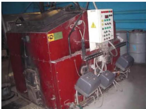
Fig. 2.4 – The IN-50 installation
