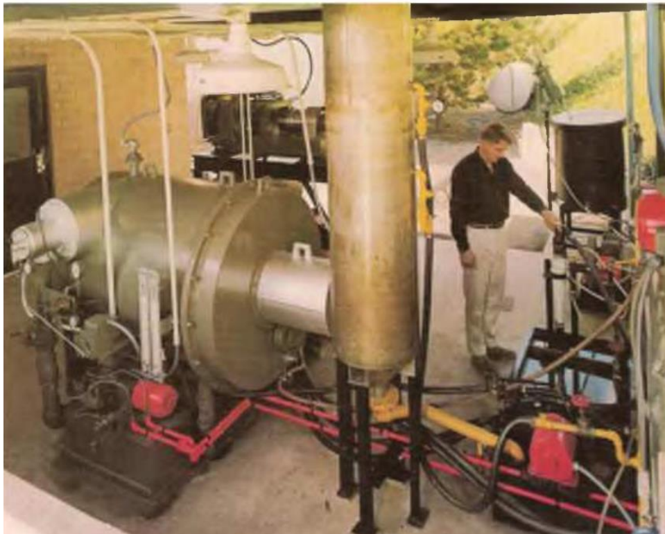
Fig. 2.9 – Horizontal cyclone reactor for the thermal treatment of sludge
